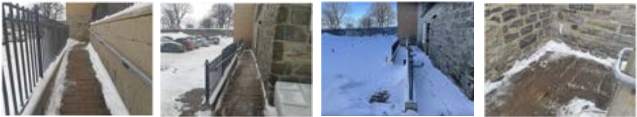
Figure 10. Images of the secondary entrance ramp
