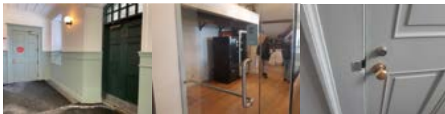
Figure 15. Images of the interior doors
