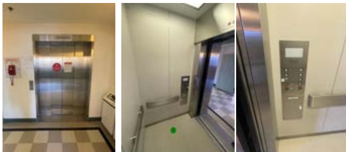
Figure 19. Images of the elevators
