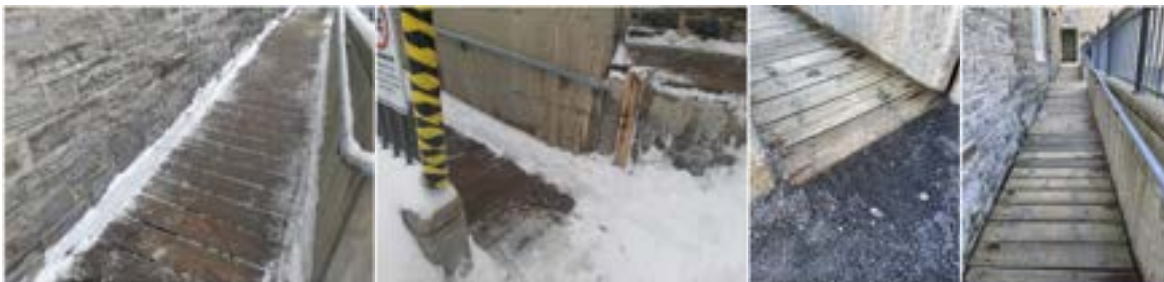
Figure 11. Images of the secondary entrance ramp
