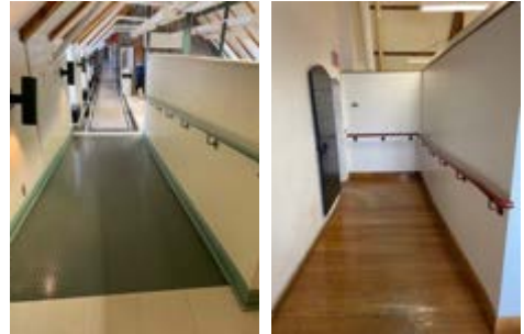
Figure 18. Images of interior railings
